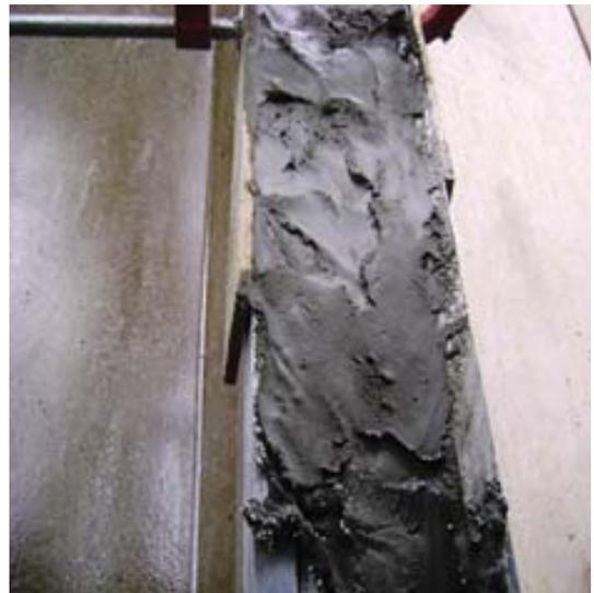
Fig. 11-Application of structural cementitious mortar for
