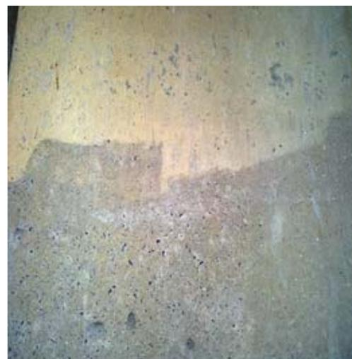
Fig. 7- Second step of cleaning: washing with pressurized water and alkaline detergent pH14.
