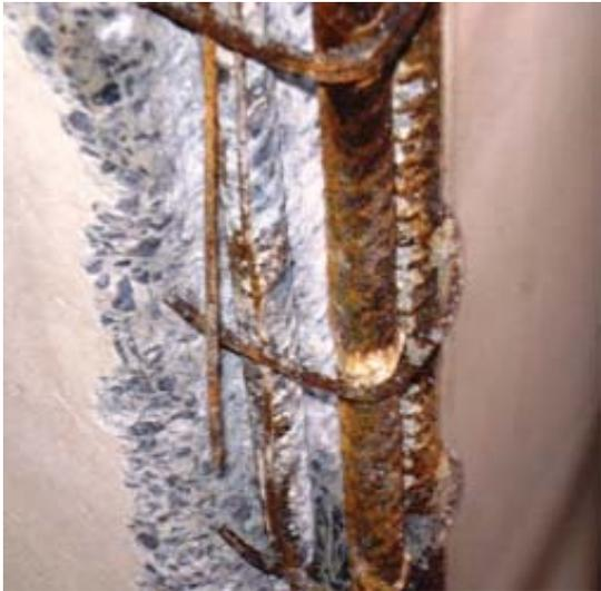
Fig. 3 High concentration of reinforcement, 4 rebar  $\theta \frac{3}{4}$  and low reinforcement coverings (6mm) The structure is already attacked by hydrochloric acid vapors.
