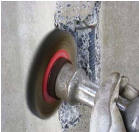
Fig. 9- Reinforcement cleaning using
