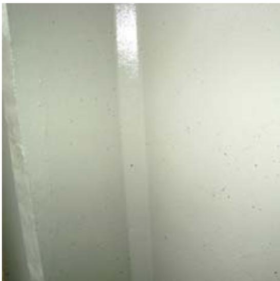
Fig. 13-Application of final coat in acrylic aliphatic polyurethane low (VOC).
