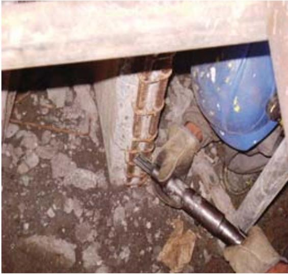
Fig. 8- Reinforcement cleaning using needle gun.
