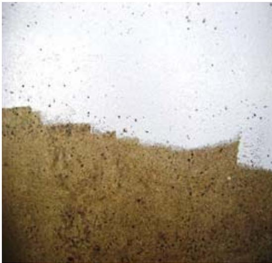
Fig. 12- Application of epoxy varnish sealer and application of intermediate coat in epoxy two component polyamide cured.
