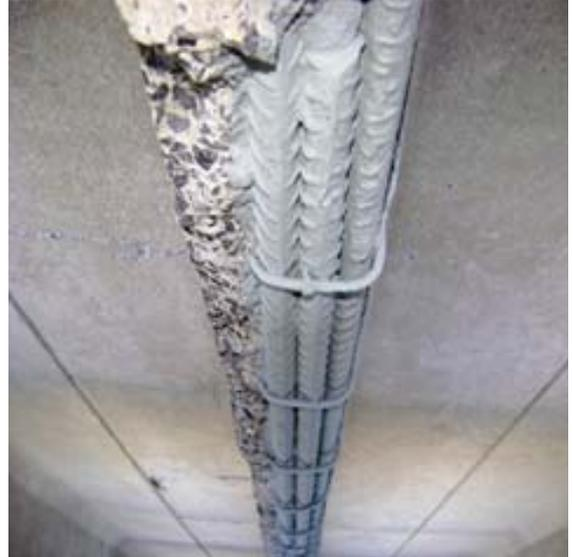
Fig. 10- Application of epoxy rich zinc for reinforcement
