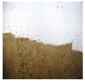
Fig. 12- Application of epoxy varnish sealer and application of intermediate coat in epoxy two component polyamide cured. Source: Setaviso Engineering [2013]
