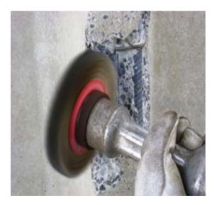
Fig. 9- Reinforcement cleaning using steel rotating brush. Source: Setaviso Engineering [2013]
