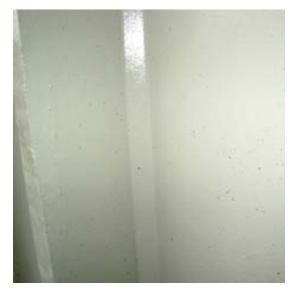
Fig. 13-Application of final coat in acrylic aliphatic polyurethane low (VOC). Source: Setaviso Engineering [2013]
