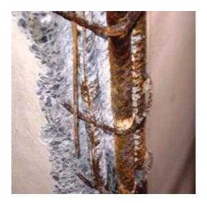
Fig. 3 High concentration of reinforcement, 4 rebar θ ¾ and low reinforcement coverings (6mm) The structure is already attacked by hydrochloric acid vapors.
