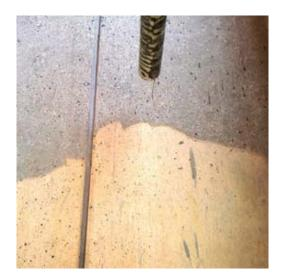
Fig. 6- First step of cleaning: washing with hot water Source: Setaviso Engineering [2013]
