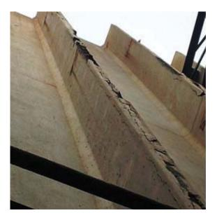
Fig. 1 Pathologies presented by fence panels . Source: Setaviso Engineering [2013]
