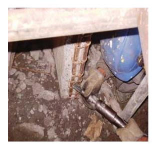
Fig. 8- Reinforcement cleaning using needle gun. Source: Setaviso Engineering [2013]
