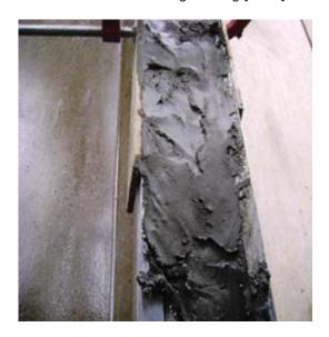
Fig. 11-Application of structural cementitious mortar for repairs up to 7cm deeper. Source: Setaviso Engineering [2013]
