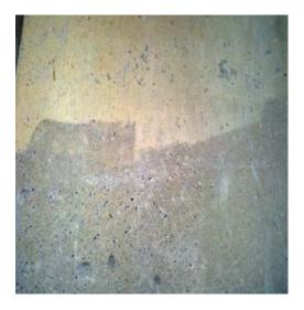
Fig. 7- Second step of cleaning: washing with pressurized water and alkaline detergent pH14. Source: Setaviso Engineering [2013]
