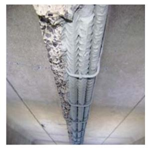
Fig. 10- Application of epoxy rich zinc for reinforcement protection. Source: Setaviso Engineering [2013]
