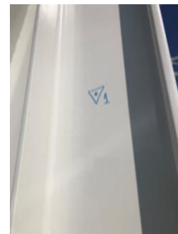
Figure 5 – Target 1 marked on a column
