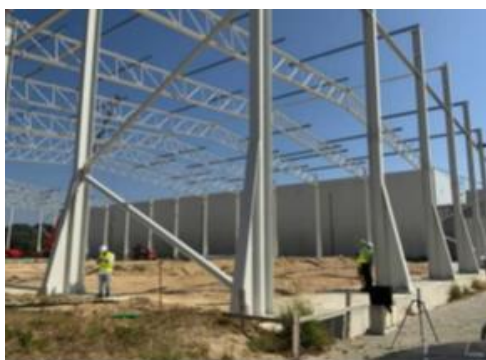
Figure 6 – Photograph of the structure with BLK 360
