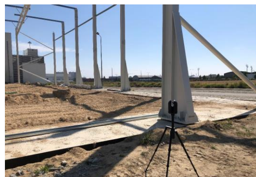
Figure 7 - Photograph of the structure with camera
