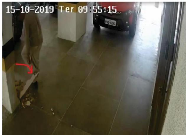
Figure 3 – Intervention made in the pillars
